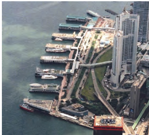
Site 1 near Central Piers No. 4-6
