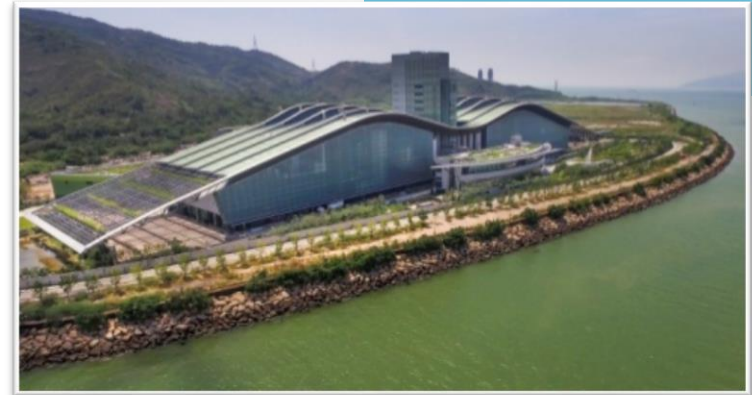
T • Park Sludge Treatment Plant
