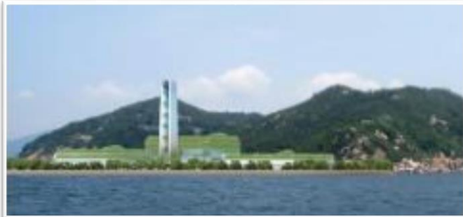
Integrated Waste Management Facility
