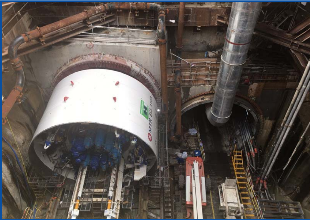
TBM mining towards Exhibition Station
