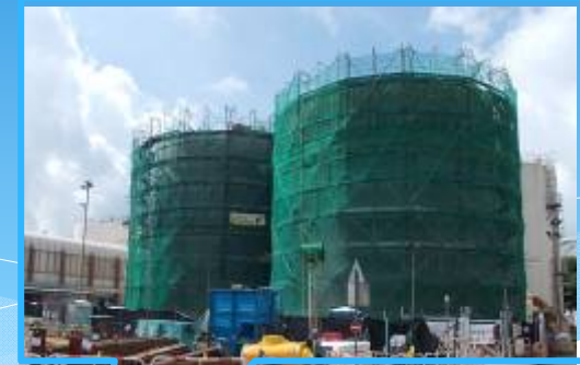
Sludge Storage tanks
