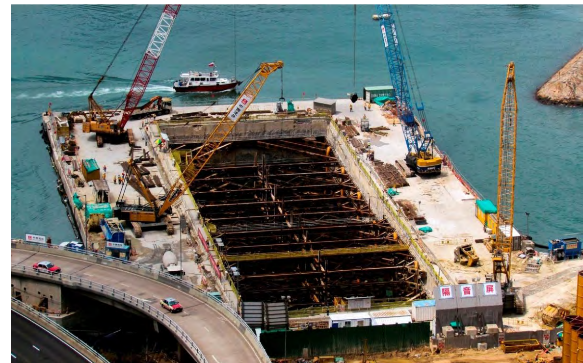
Figure 4-5 – Temporary Reclamation of Central-Wan Chai Bypass
