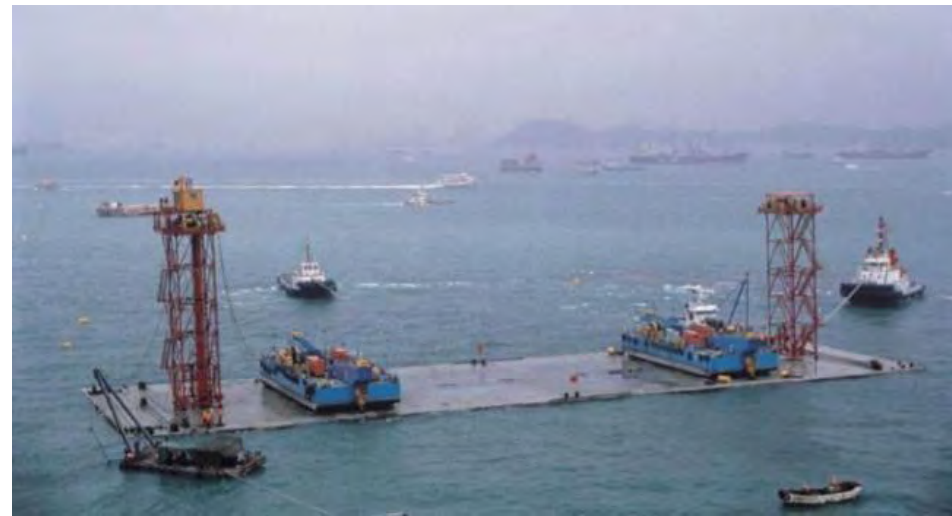
Figure 3-5 – Example of Immersed Tube Tunnel (IMT)
