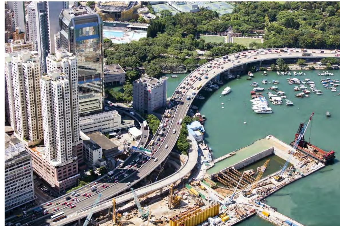
Figure 4-4 – Temporary Reclamation of Central-Wan Chai Bypass
