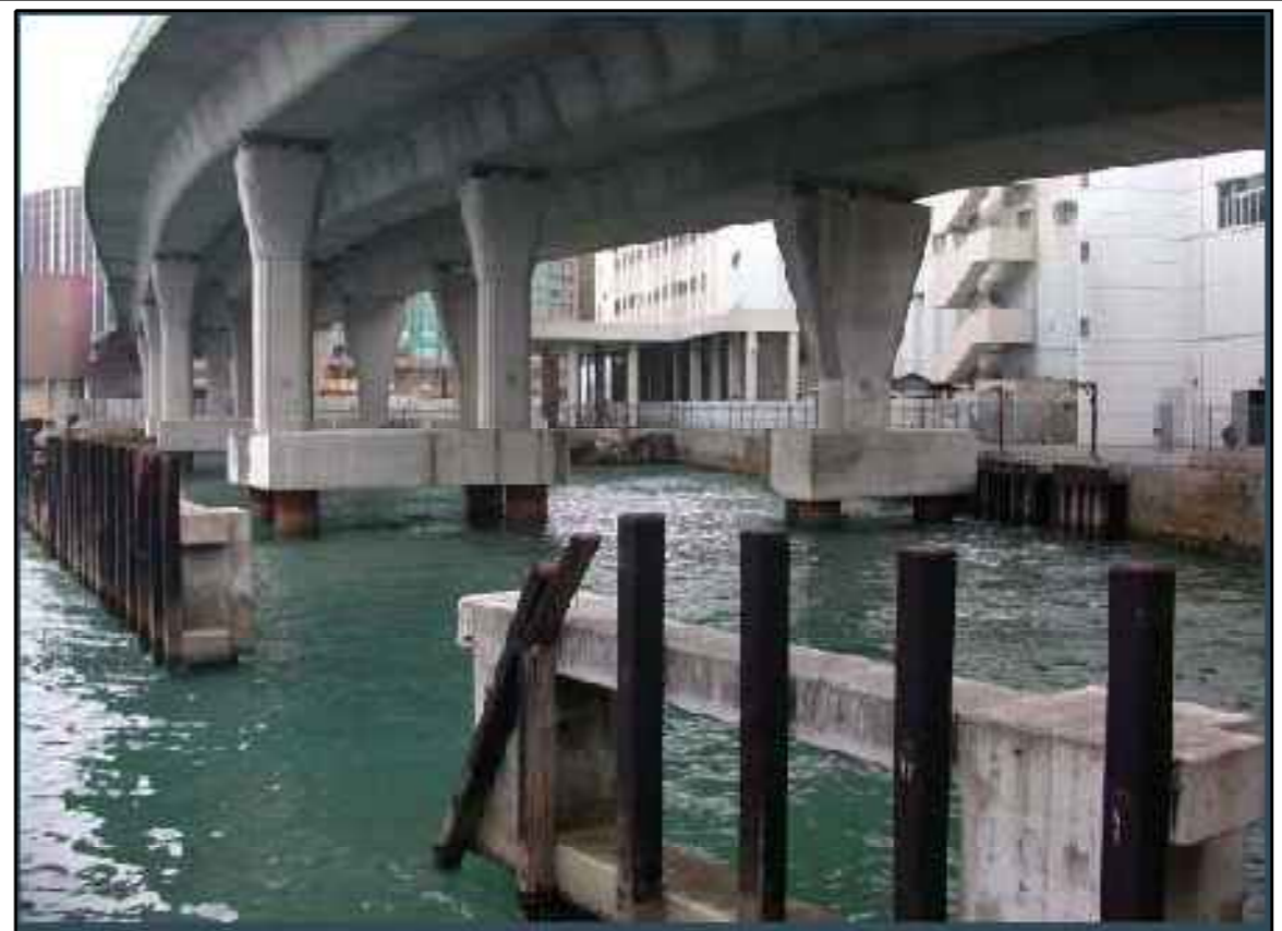
HUNG HOM BYPASS FENDER PILES TO BE REINSTATED
