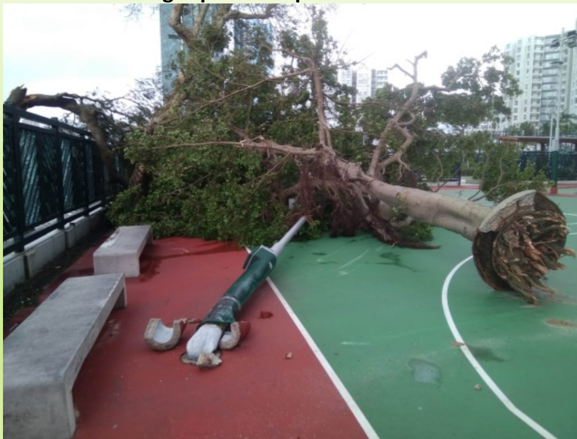
Tree and light pole collapsed 燈柱及樹木倒塌
