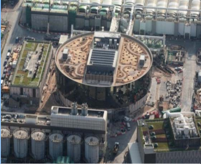
World's Largest Chemically Enhanced Primary Treatment Plant
