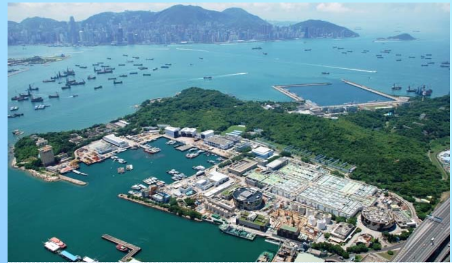
Hong Kong's Largest Ever Environmental Infrastructure Project
