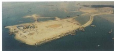
Aerial view of construction in April 1997.
