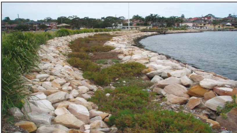
← Kogarah Bay, Australia A step-type seawall with a bench of saltmarsh vegetation
