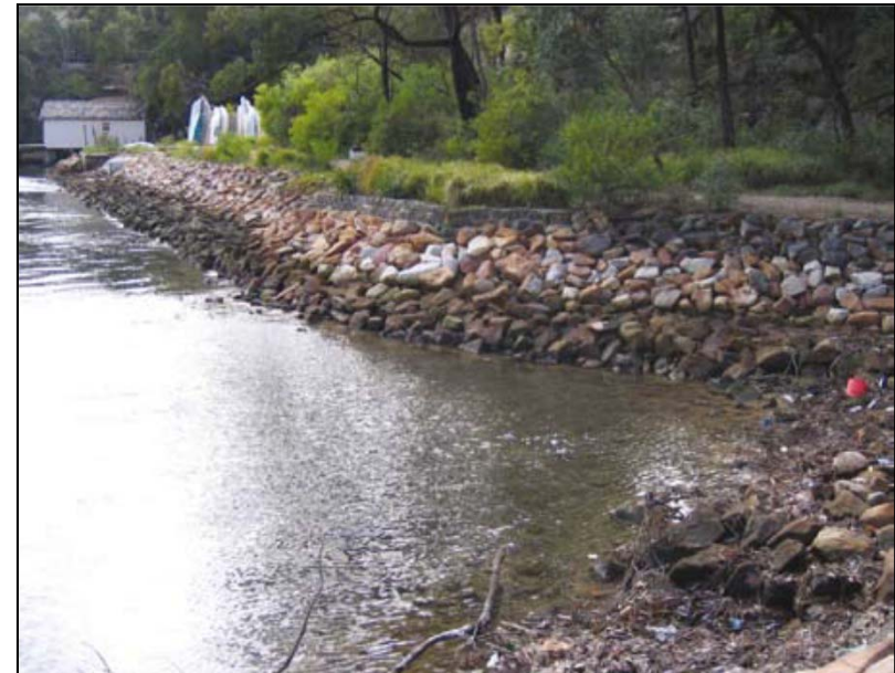
Quakers Hat Bay, Sydney, Australia → Boulders have been added to the front of seawall to improve total habitat surface area
