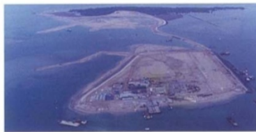
A view of Pulau Sakeng in October 1996 shows the island enlarged to house the future landfill facilities.
