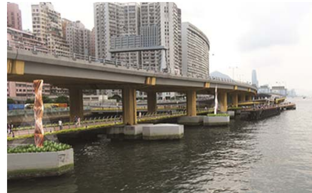
Boardwalk underneath IEC
