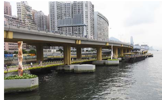
Boardwalk underneath IEC
