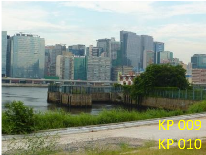
Kai Tak Fire Boat Landing No. 1 & 2 [abandoned]
