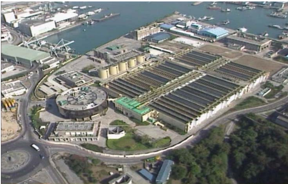
Figure 2 – Stonecutters Island Sewage Treatment Works in 2001
