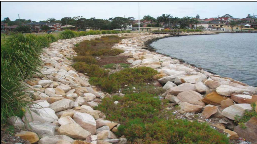
← Kogarah Bay, Australia A step-type seawall with a bench of saltmarsh vegetation
