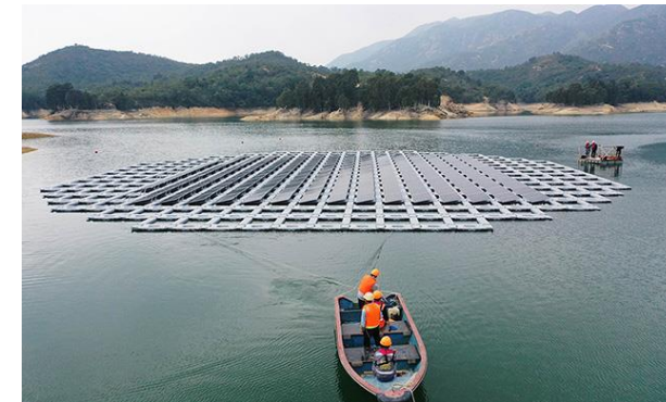
Tai Lam Chung Reservoir
