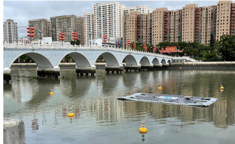
Mock-up in Shing Mun River
