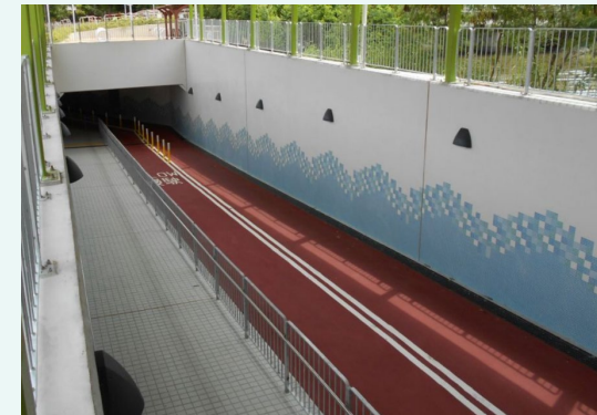
Reference of existing cycle track and footpath subway
