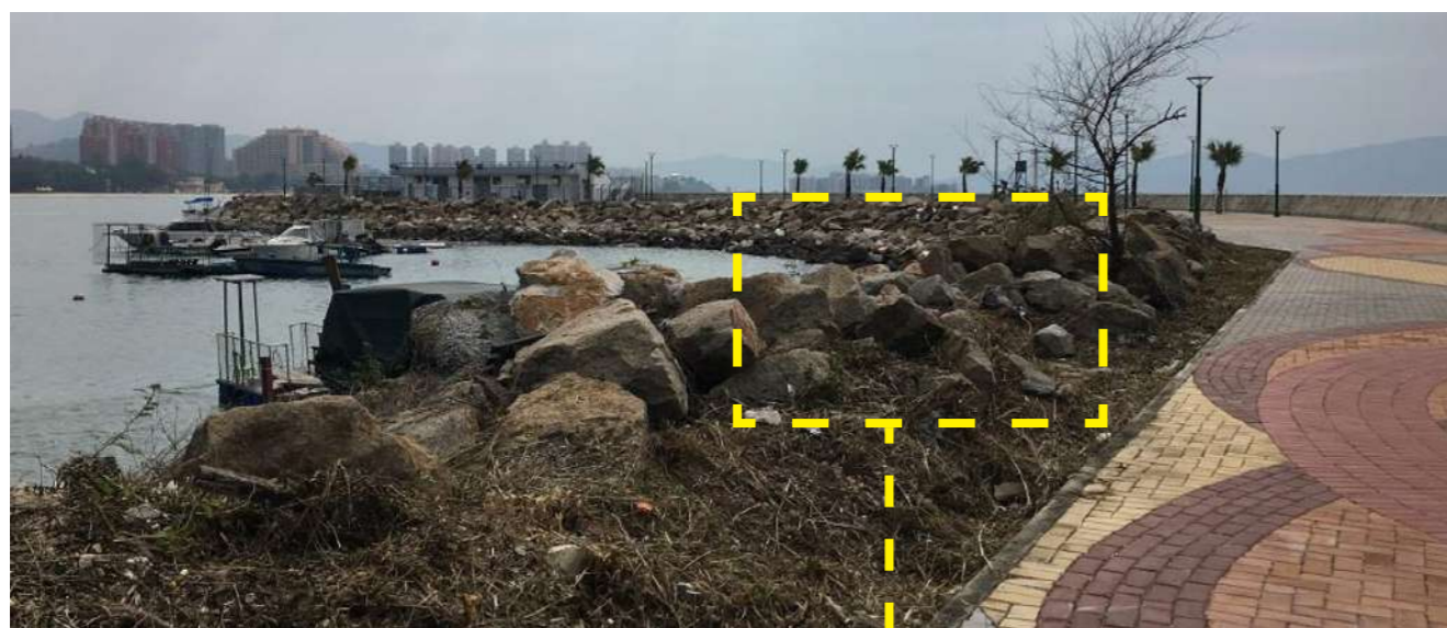
Gentle slope formed of big rocks as buffer zone between walking path and water
