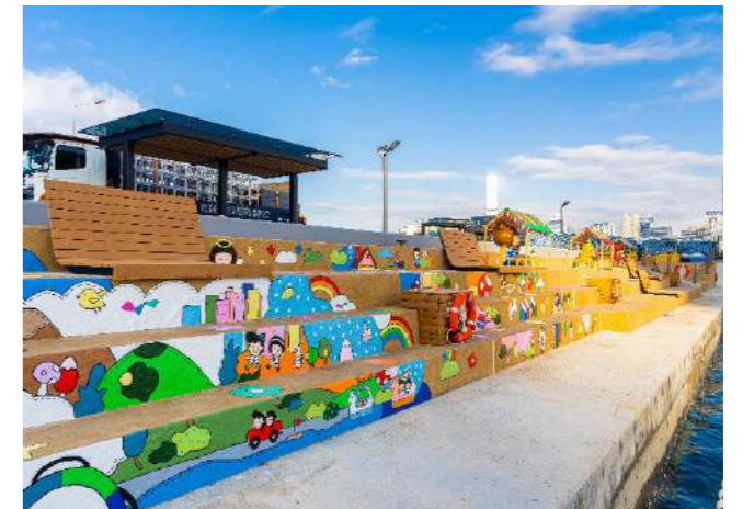
@ Water Sports and Recreation Precinct (Phase 2)
