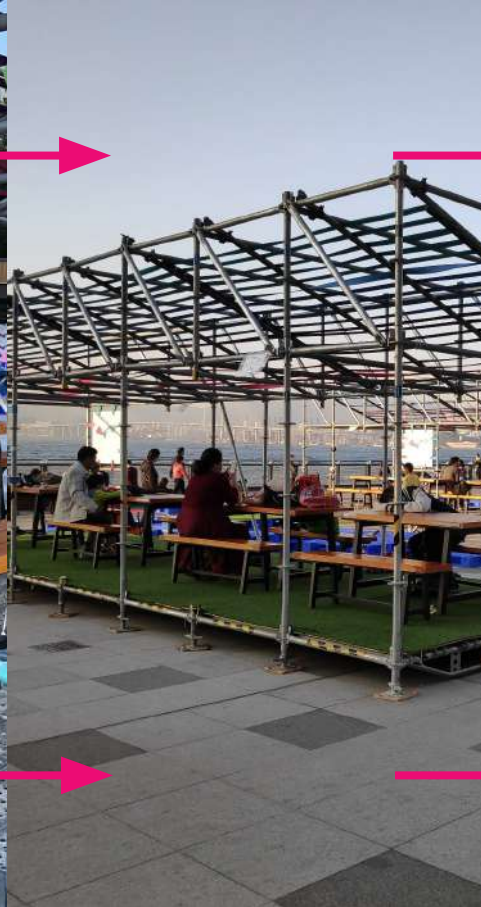
Artificial turf is added to the ground plate
