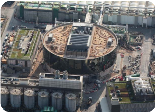
Figure 8 – New Main Pumping Station
