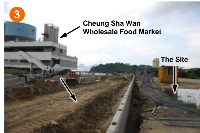
A Planned 25m-wide Pedestrian Walkway (Under Construction)
