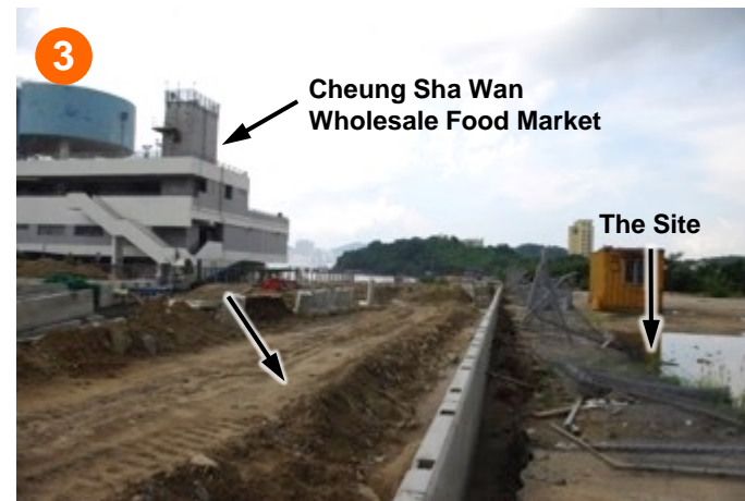
A Planned 25m-wide Pedestrian Walkway (Under Construction)
