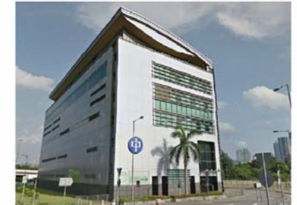
5. CLP CENTENARY SUBSTATION
