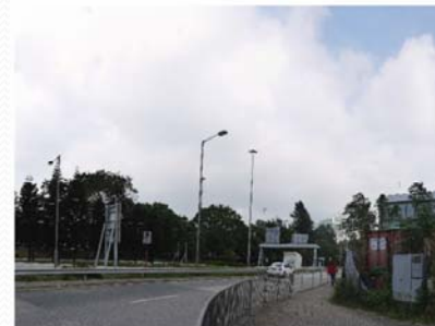
3. VIEW TOWARDS W KOWLOON HIGHWAY
