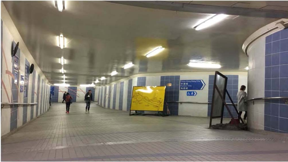
INTERIOR OF EXISTING PEDESTRIAN SUBWAY - EXISTING CONDITION
