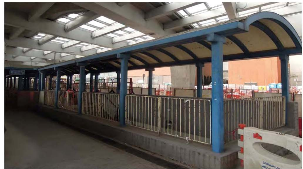
EXISTING PEDESTRIAN SUBWAY ENTRANCE AT XIQU CENTRE - EXISTING CONDITION
