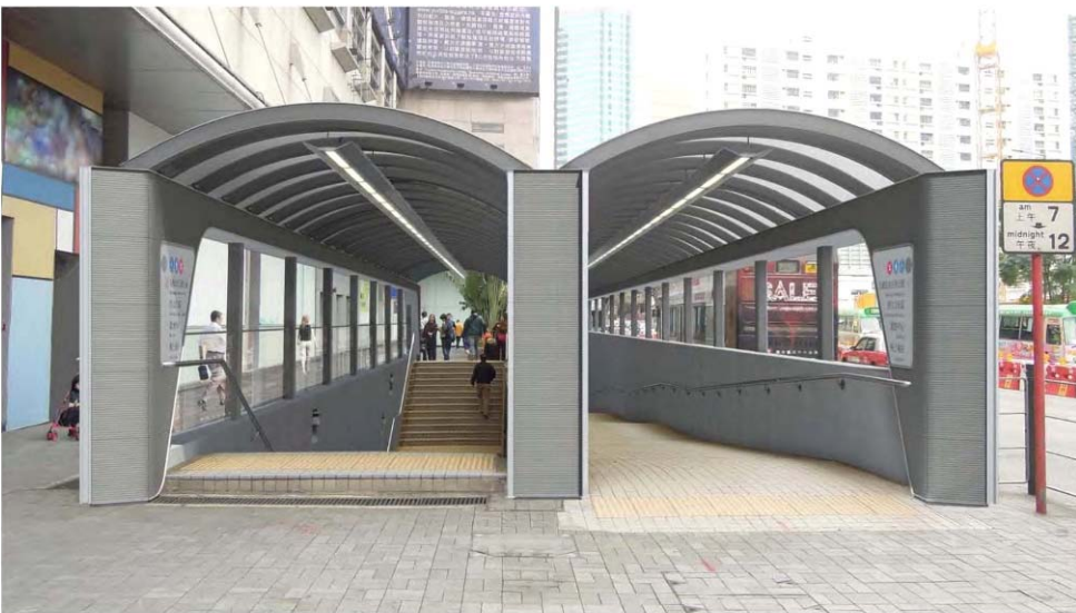
EXISTING PEDESTRIAN SUBWAY ENTRANCE NEAR THE VICTORIA TOWER - AFTER BEAUTIFICATION WORKS
