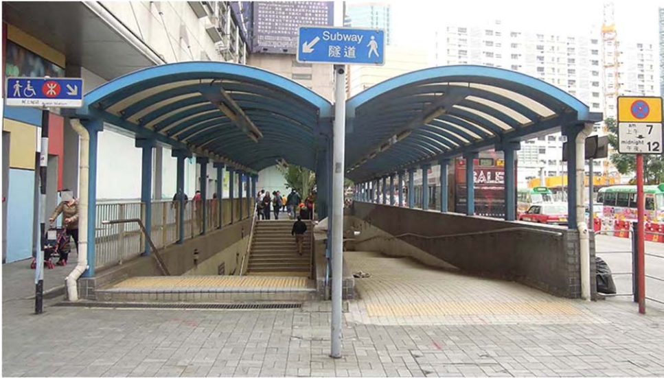
EXISTING PEDESTRIAN SUBWAY ENTRANCE NEAR THE VICTORIA TOWER - EXISTING CONDITION
