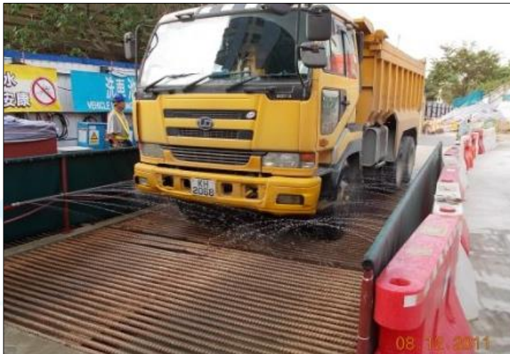
Provide wheel-washing facility at site entrance
