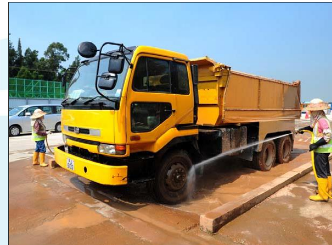
Provide wheel-washing facility at site entrance
