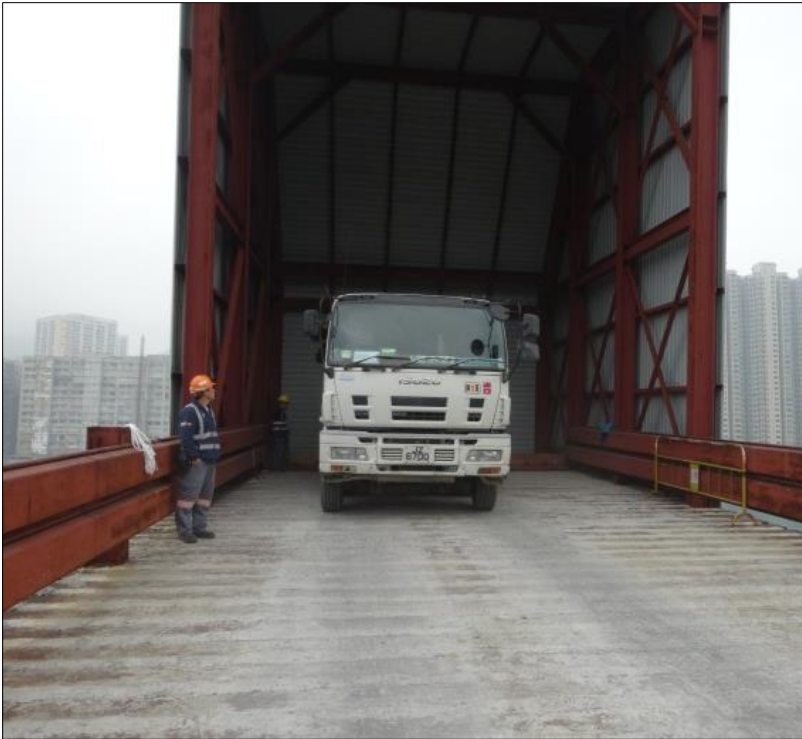
Dust enclosure with sprinkler system for temporary barging facility
