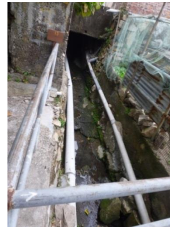
Existing Surface Channel
