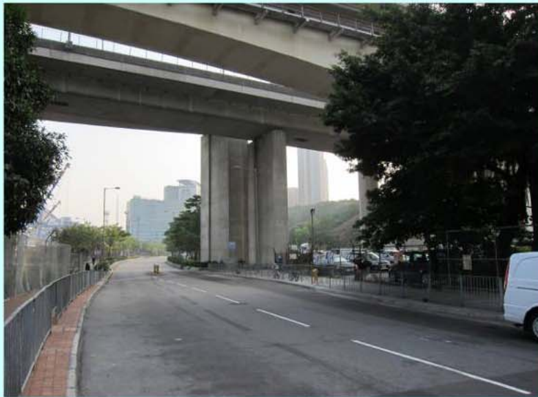
Photo 6: Beneath of Kwai Tsing Bridge.
