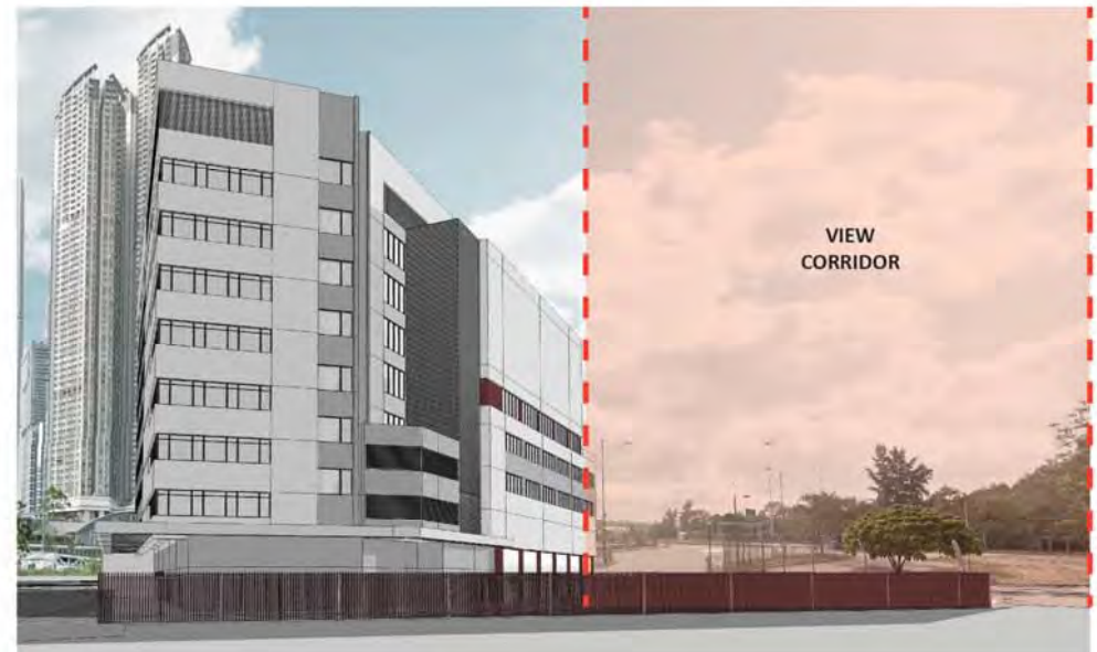
VIEW FROM LIN CHEUNG ROAD
