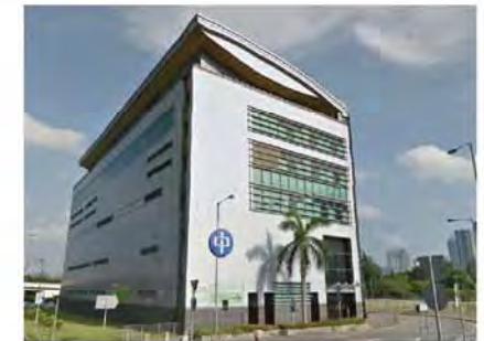
5. CLP CENTENARY SUBSTATION
