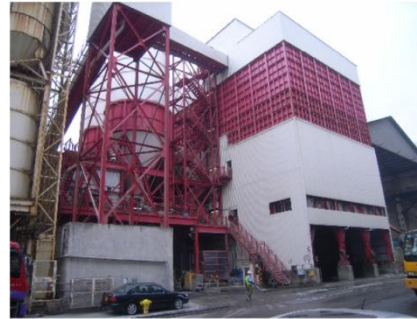
混凝土配料廠 CONCRETE BATCHING PLANT
