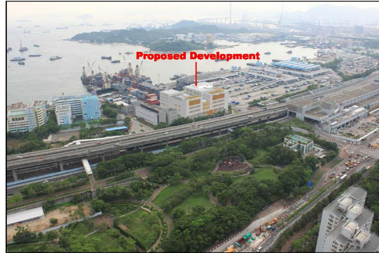
VP2 Metro Harbour View, Top Level, Unmitigated
