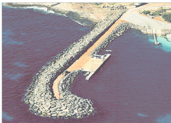
Photo 3: Example of rubble mound breakwaters
