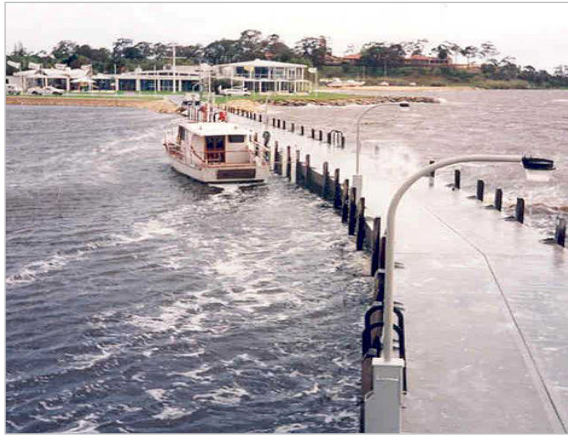
Photo 4: Example of pile supported structural breakwater
