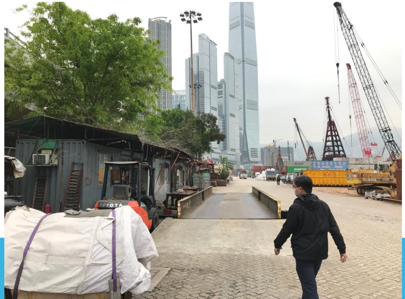
Weight Bridge and Access Road
