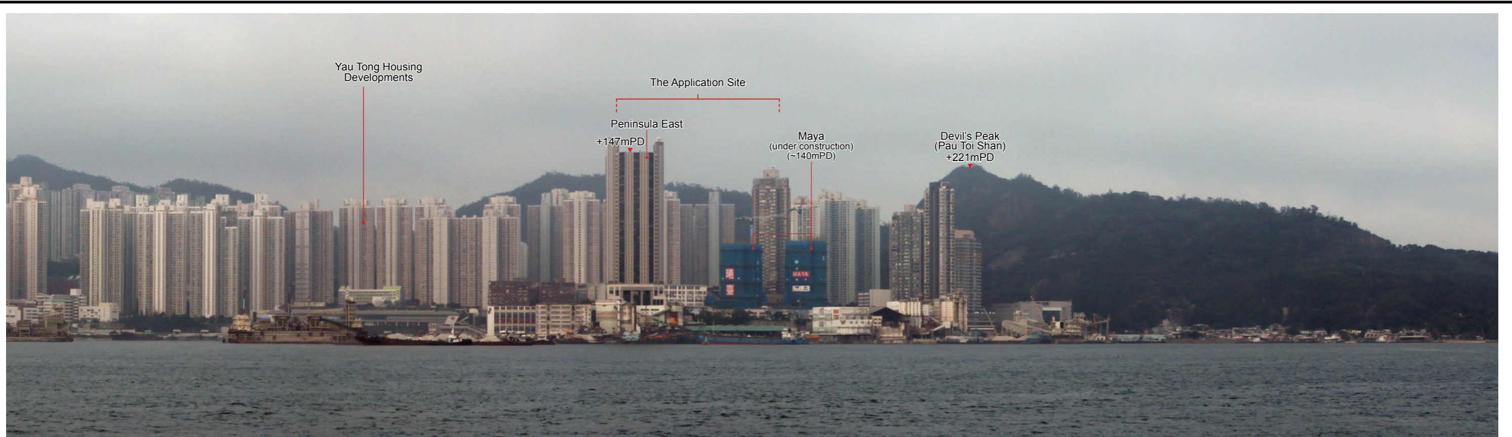
Existing View (March 2019)
