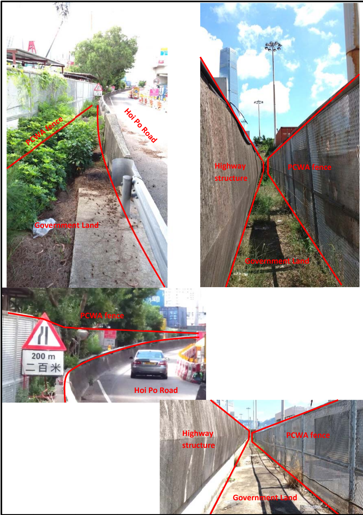
Figure 5b. Photos showing the available Government Land along Hoi Po Road, between the layby and Hoi Fai Road, pinch point about 0.5 metre wide.
