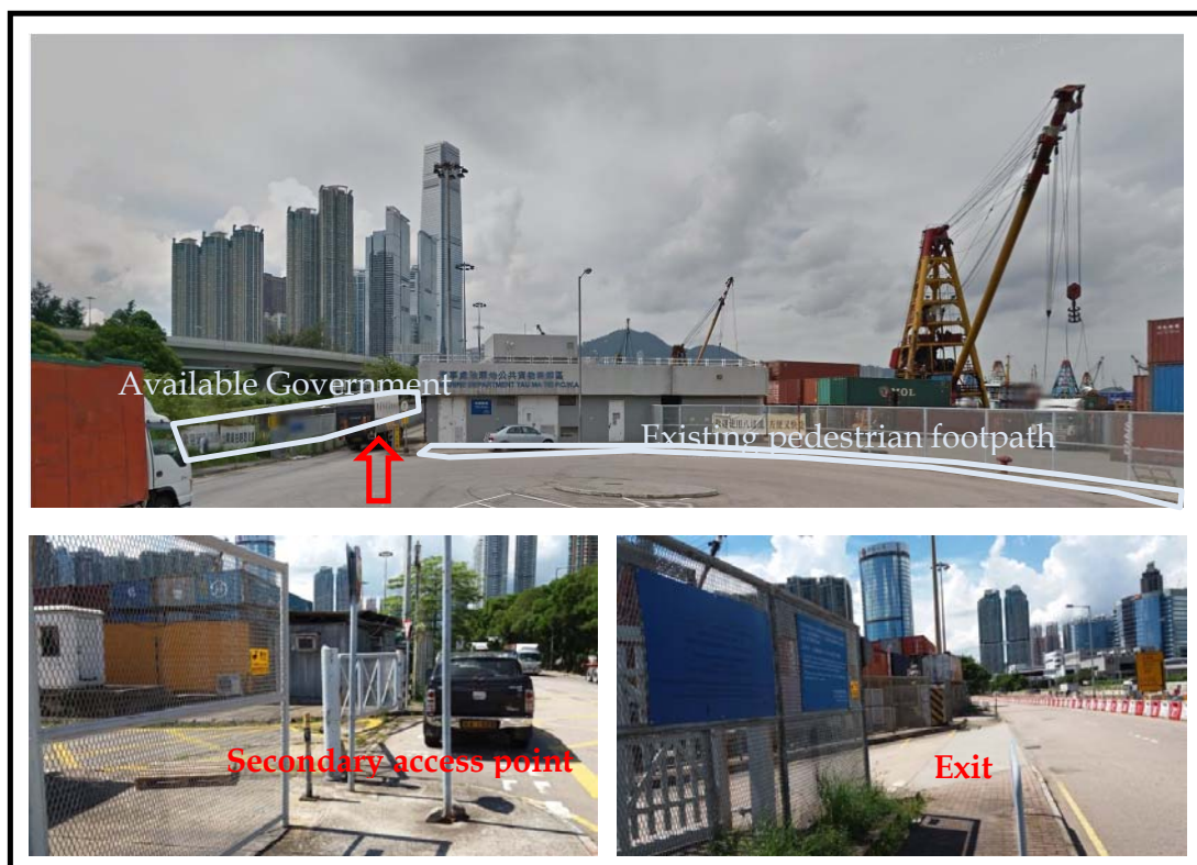
Figure 4. Photos showing the vehicular access points on Hoi Fai Road.
