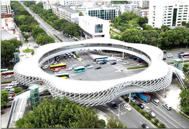
Figure 9c. Chunhua footbridge in ShenZhen with bays. Source: http://www.arch2o.com
