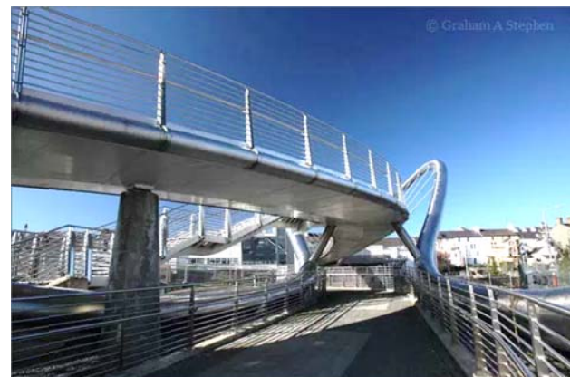
Figure 9f. Celtic gateway bridge in UK, in levels. Source: https://geotopoi.files.wordpress.com
