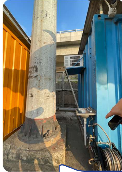
High Mast Light with Massive Footing
