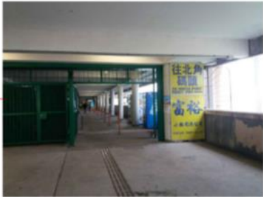
Existing Pier Canopy (Outside Site Boundary): To be demolished by others
