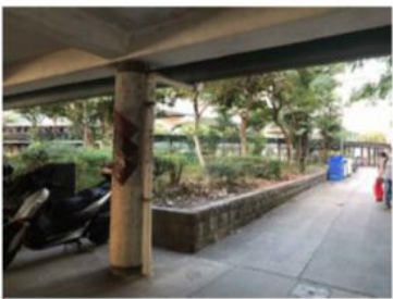
Existing Planter: To be retained
