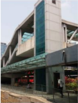
Existing Covered Walkway: Proposed covered walkway to be connected to the existing covered walkway
