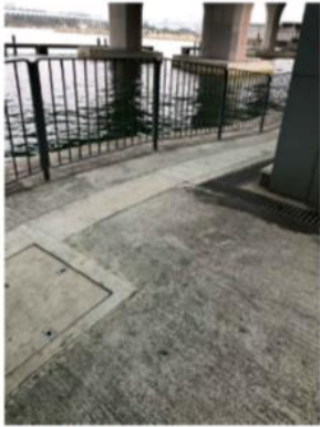
Existing Sloped Walkway: Modification of slope
