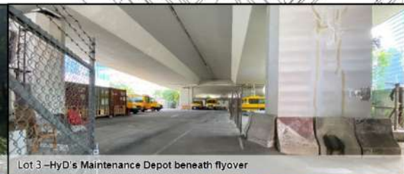
Lot 3 – HyD's Maintenance Depot beneath flyover
