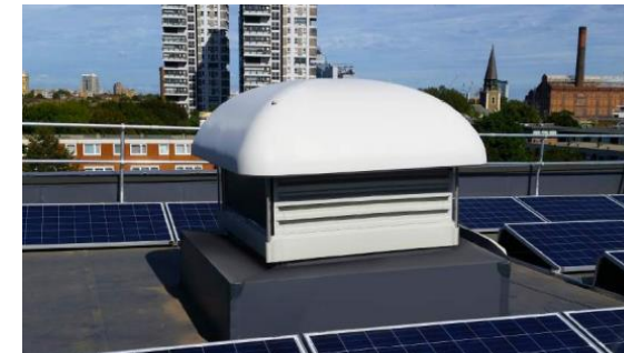
Supplier: Monodraught – X-Air Thermal Mixing Unit
