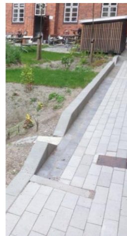
Proposed openings at kerb for rainwater runoff
