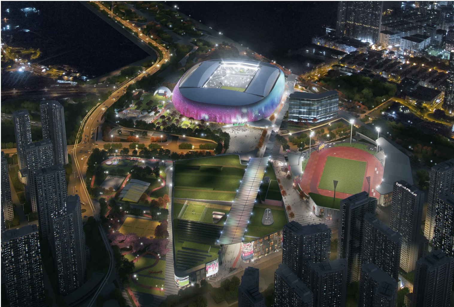
Overall View – night time
