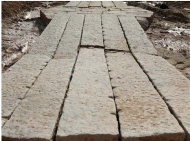
Granite Deck of the LTSB
