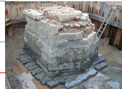
Remnant of Supporting Pillar Section
