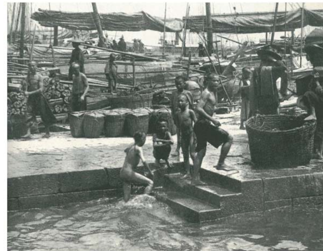
Landing Platform of a Sheung Wan Pier
