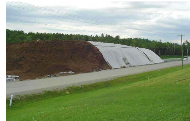
Cover temporary stockpile of excavated materials with impervious sheets
