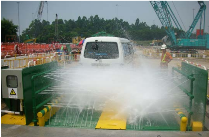
Wheel-washing facility at site entrance
