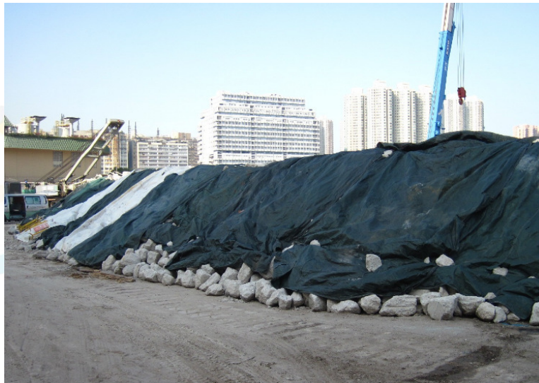
Dust enclosure with sprinkler system
