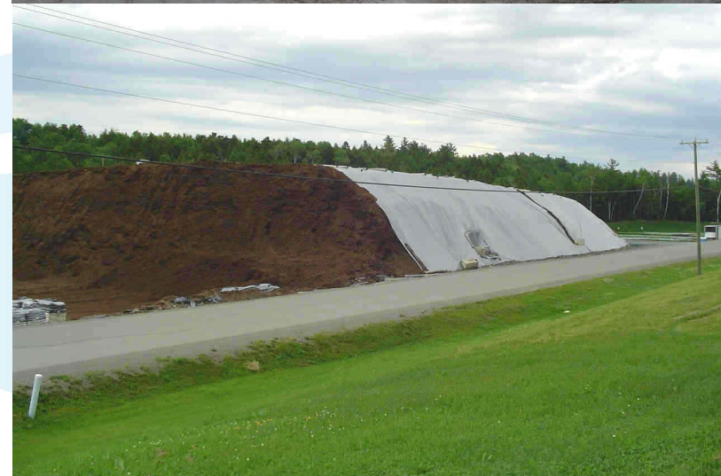
Cover temporary stockpile of excavated materials with impervious sheets
