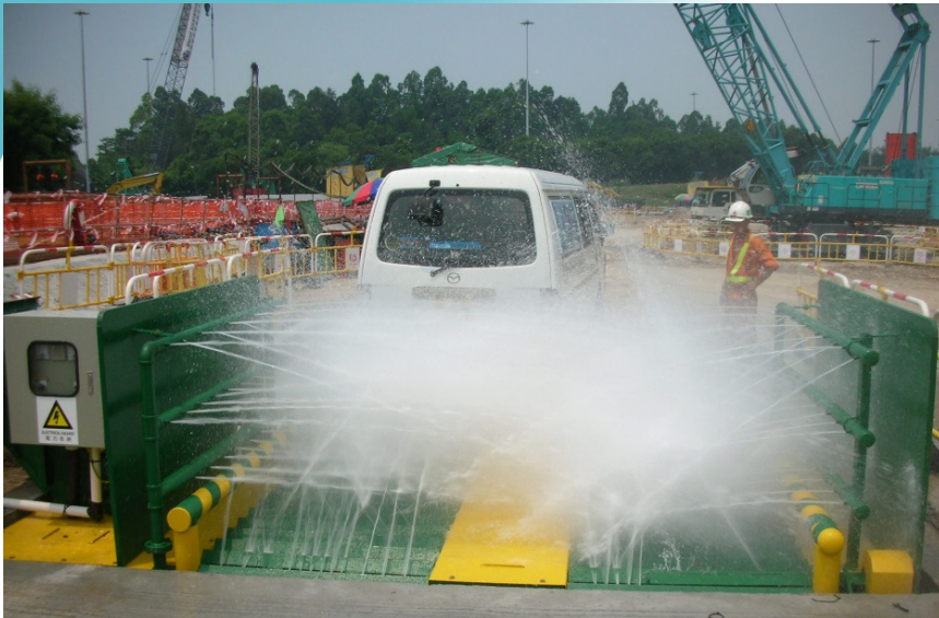
Wheel-washing facility at site entrance
