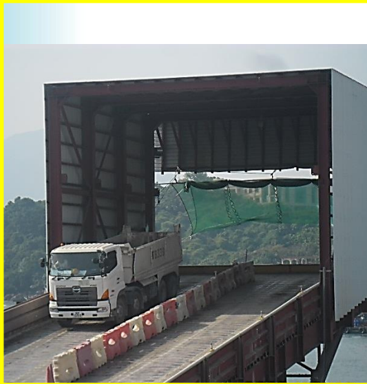
Dust enclosure with sprinkler system
