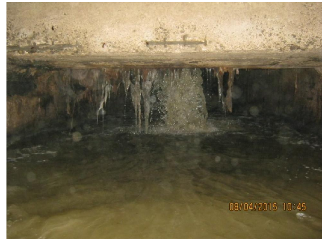
Polluted flow to stormwater drainage system from damaged sewers / sewerage manholes
