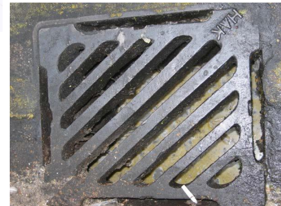
Illegal discharge of polluted flow to road side gullies
