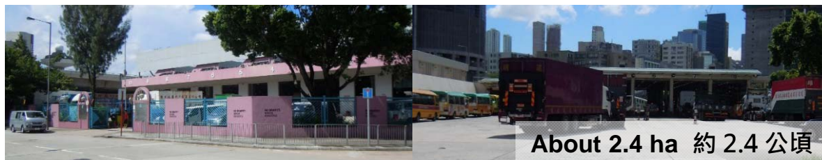
TD's Vehicle Examination Centres 運輸署的驗車中心
