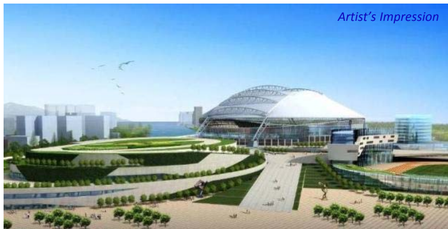
Multi-purpose Sports Complex (MPSC)
