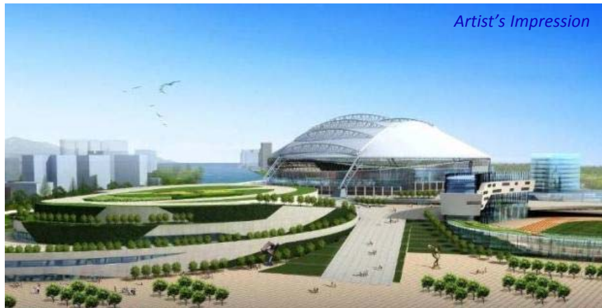
Multi-purpose Sports Complex (MPSC)
