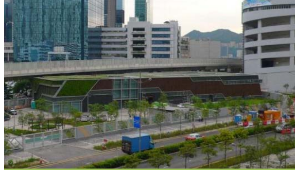
District Cooling System (Phase I)
