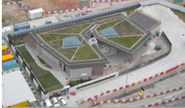
Sewage Pumping Station
