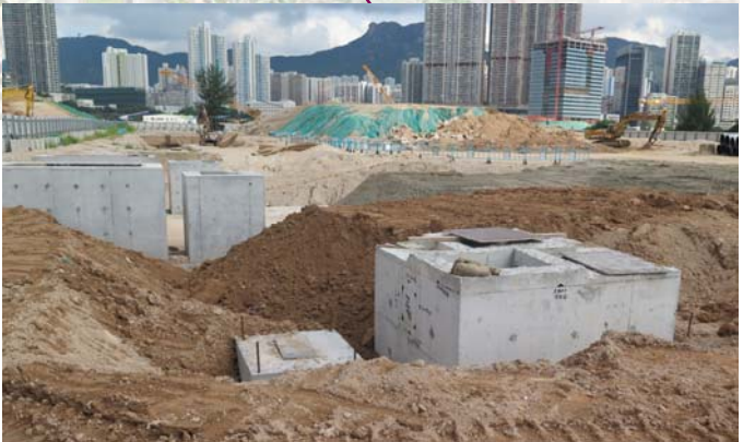
Stage 4 Works (To be completed in end 2016)
