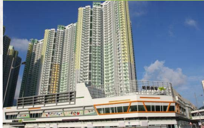
Public Rental Housing – Kai Ching / Tak Long Estate
