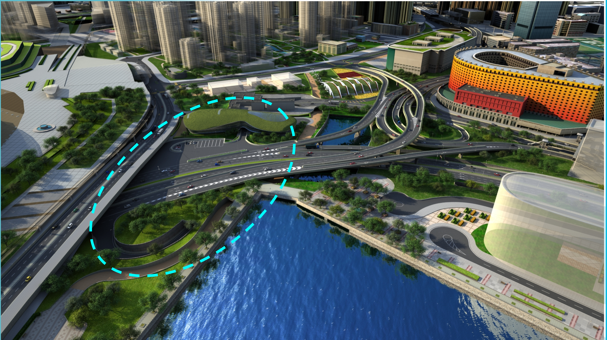
Pedestrian Access to Kai Tak Promenade
