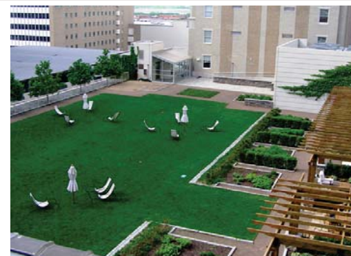
07 綠化屋頂 Accessible Green Roof
