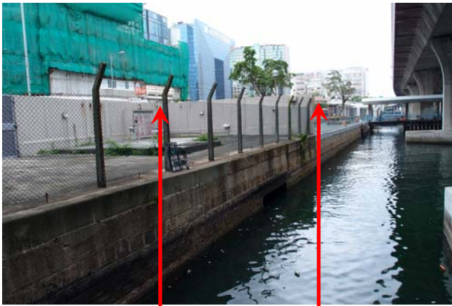
DWFI at Tsun Yip Street
