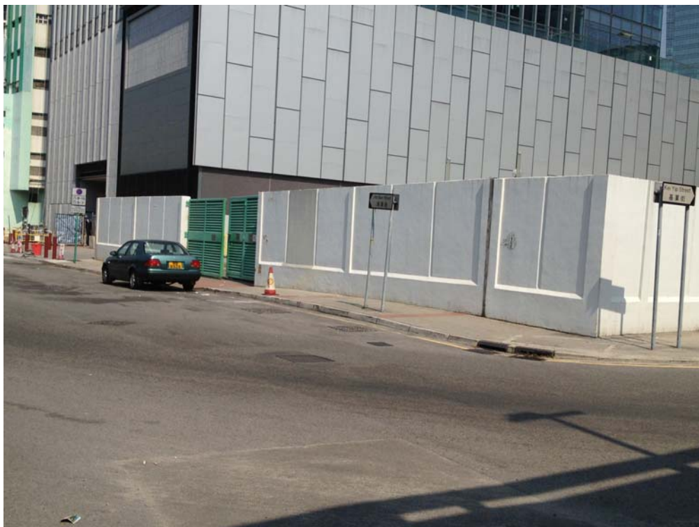
Beautification of Intermediate Sewage Pumping Station at Kei Yip Street
