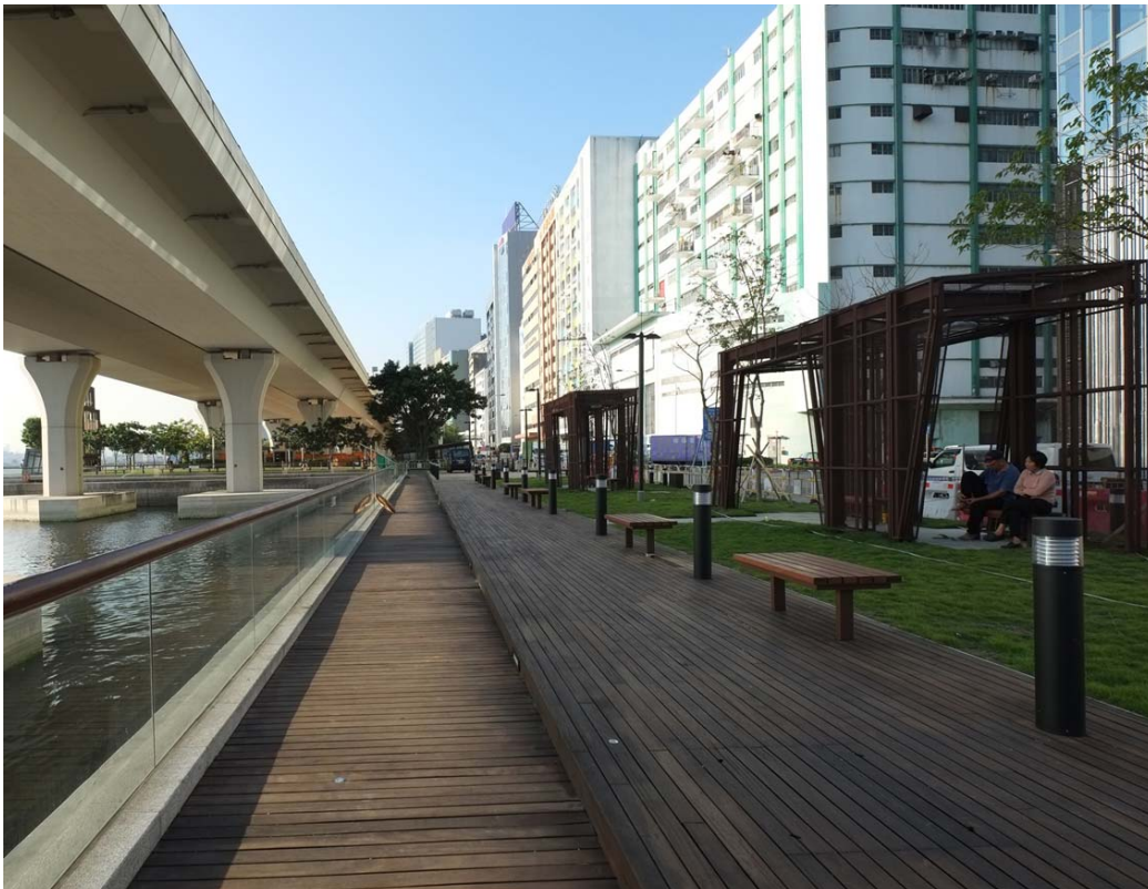
Improvement of Hoi Bun Road Sitting-out Area
