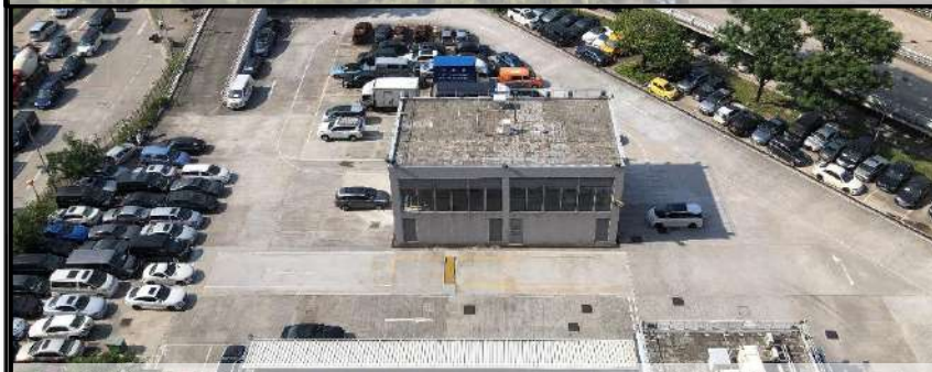
Lot 1 – Police Vehicle Examination and Detention Centre
