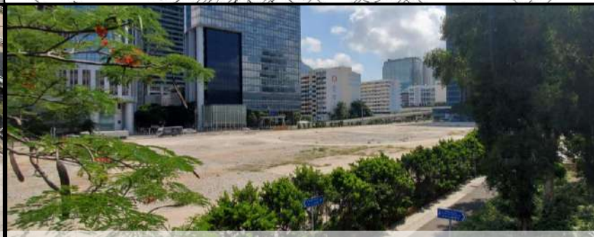
Lot 2 – Former EPD's Waste Recycling Centre
