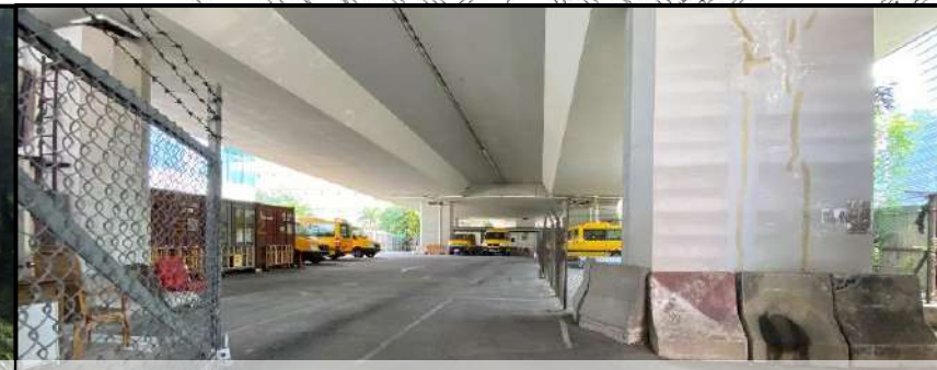
Lot 3 – HyD's Maintenance Depot beneath flyover
