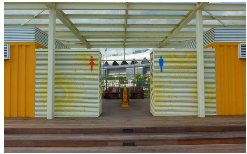
Adoption of “Energy Swirl” graphic on the façade of main entrance of temporary toilets at Shing Fung Road Station
